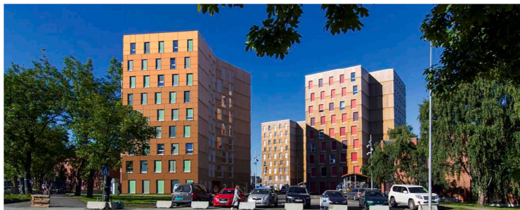
Fig. 36. FIPV renovation design proposal with monochromatic NCS colours in hue Y30R, chromaticness = 30%.
