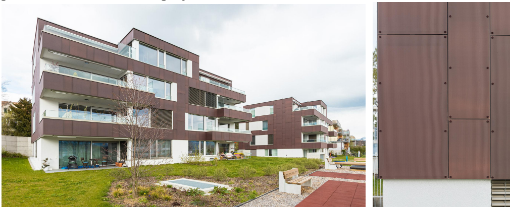
Figure 2.22: Left: Perspective view of SUNCOL Männedorf project; Right: FIPV façade details. From Sunage SA (2022) 18
