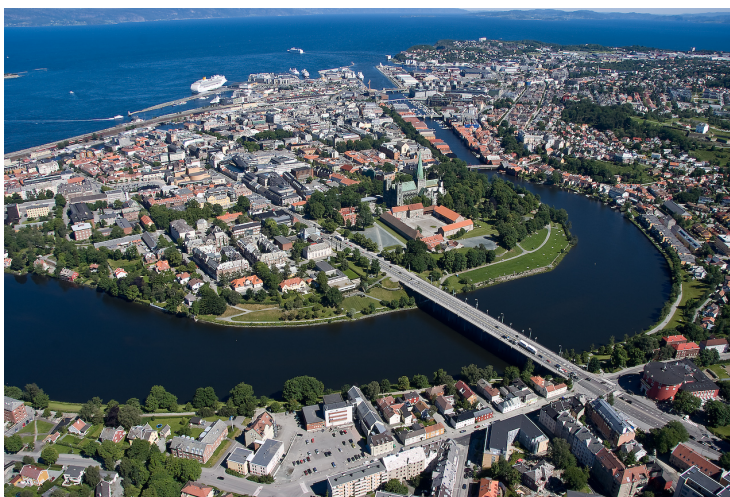
Figure 3.4: Aerial view of Trondheim city 24
