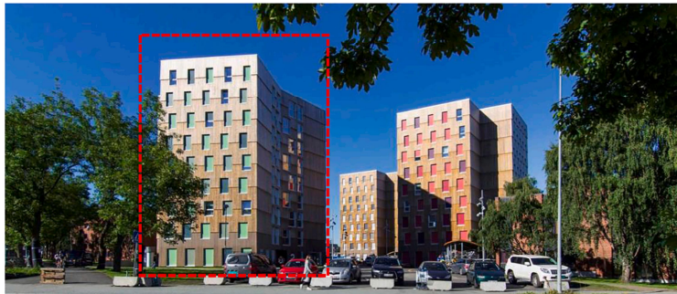
Fig. 35. Moholt student apartment tower in Trondheim. Source: www.archdaily.com .
