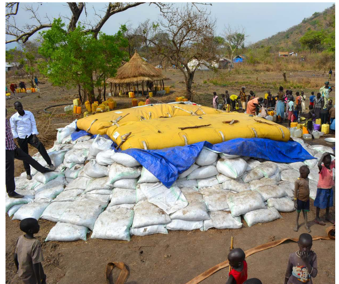
Figure 20 : A water bladder used to store water delivered by water truck in Nyumanzi 1
