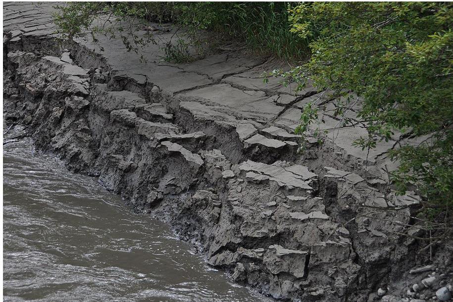
Fig. 12 Photograph of a sediment slide at the bank of the Bodendorf reservoir
