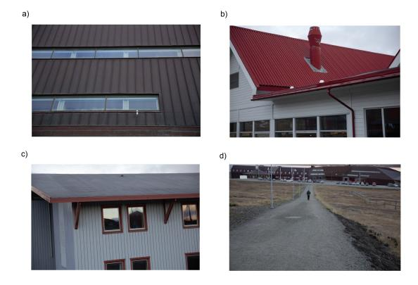
**Figure 2.** Examples for roof and road types considered in Lu et al. [54] for Longyearbyen (object ID in ()): (a) pitched metal roof, dark paint (#1); (b) pitched metal roof, red paint (#5); (c) pitched with roofing felt (#15); and (d) gravel footpath (#21).
