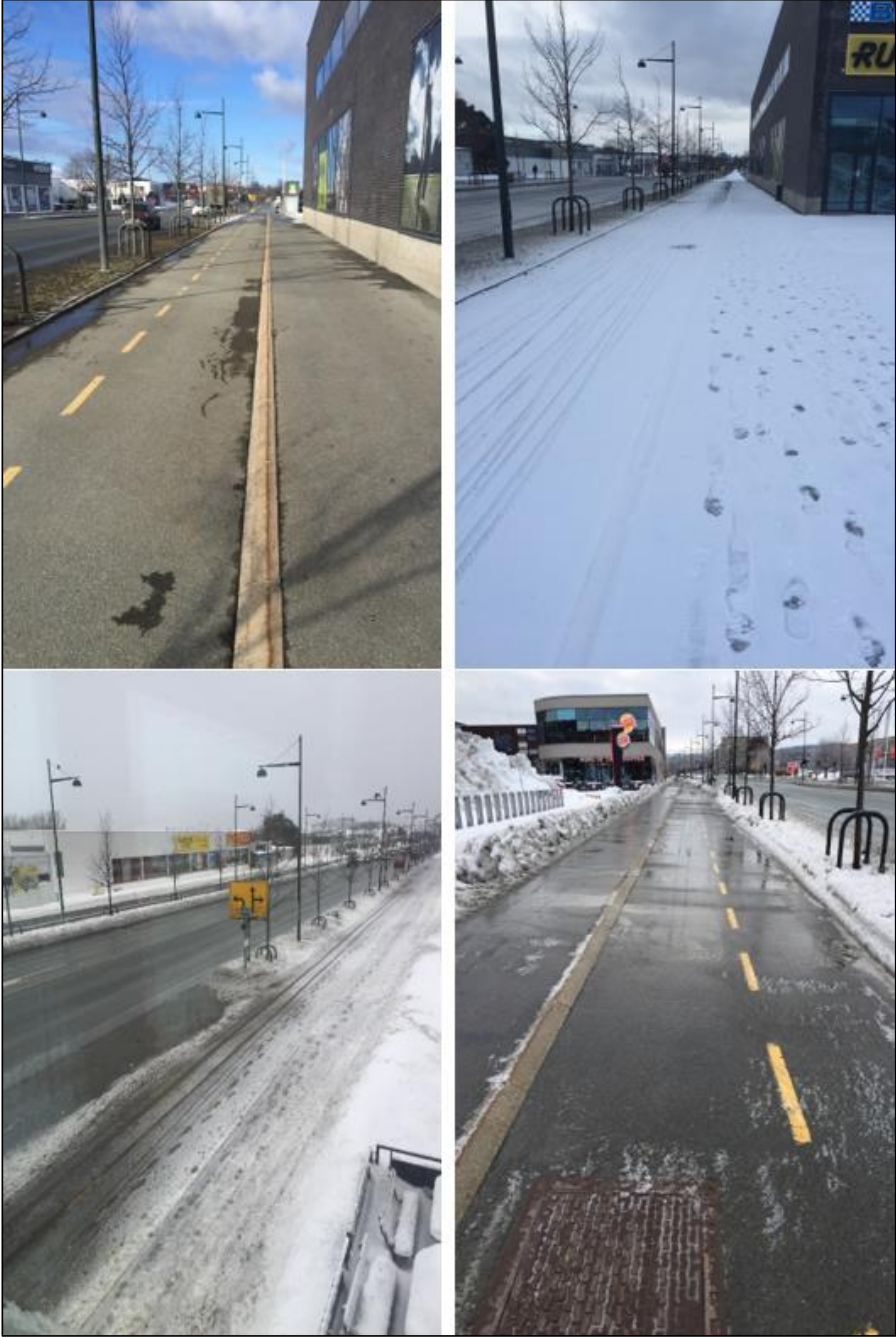
Figure 2 Typical examples of the categorized surface conditions. Top left: Bare pavement. Top right: Snow-covered pavement. Bottom left: Slush-covered pavement. Bottom right: Partly ice-covered pavement.
