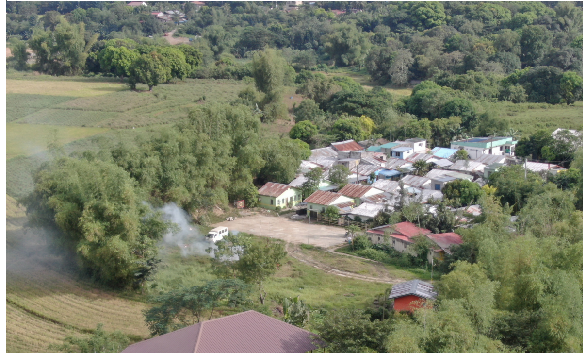
↑ Aerial view of GK Enchanted Farm. Each house is shared by two families. The row of houses was built collaboratively by the whole village through bayanihan .
