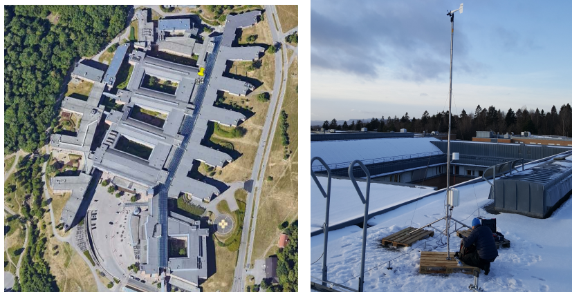
(a) Oslo University Hospital with measurement location marked (b) Experimental measurements at 6m above building D4
