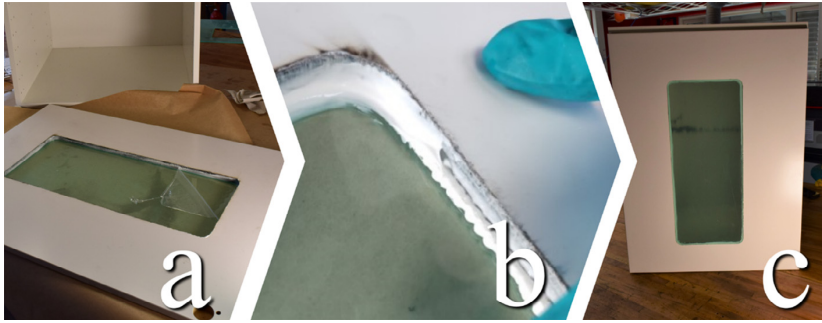
Fig. 9. a) Remove the protective film. b) Apply glue along the edge and smooth out. c) Finished installing.
