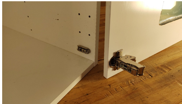
Fig. 10. Hinges installed on door.
