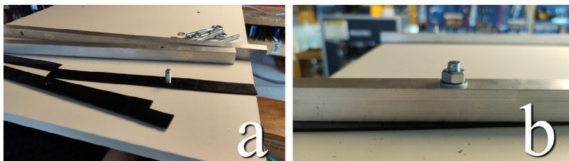
Fig. 16. a) Gasket material is cut in strips and punctured to allow eyebolts to pass through. b) Gasket, aluminum bar, eyebolt, washer, and nut fully assembled.
