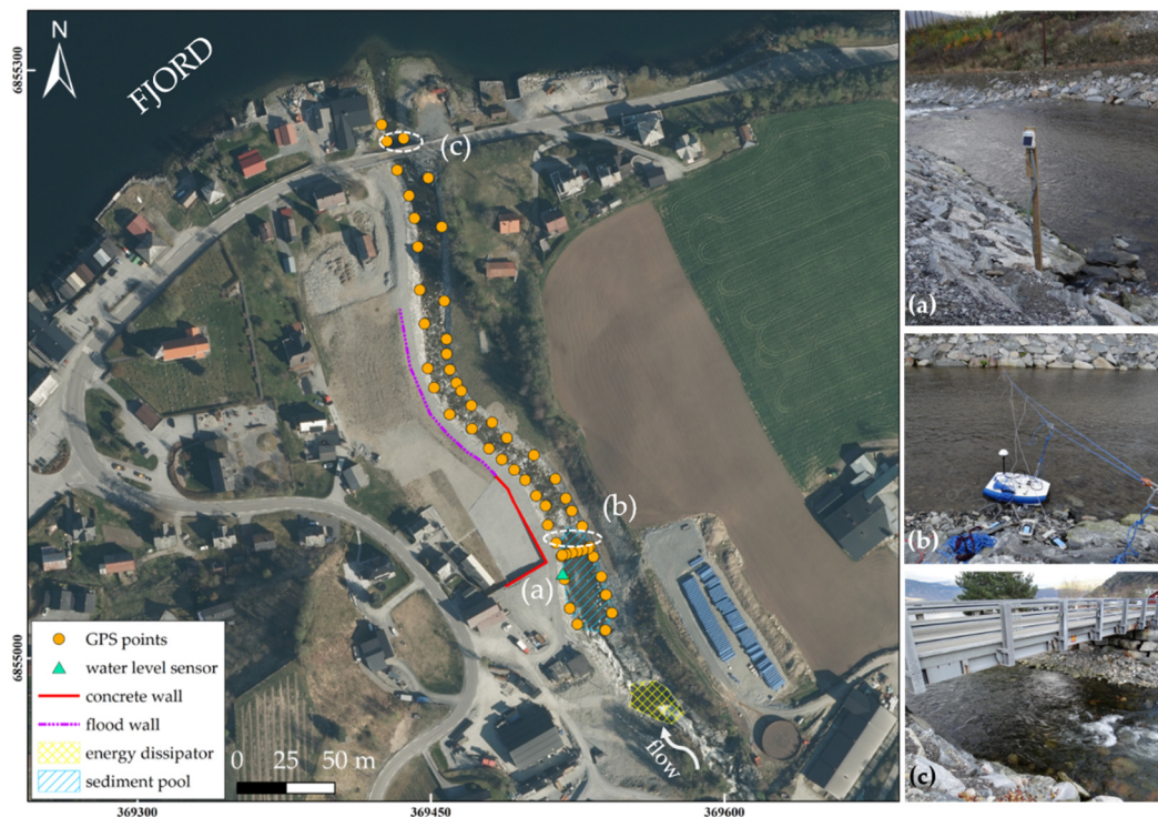
Figure 8. Flood protections and field survey in the restored the Storelva river in Utvik; (a) pressure transducer installed by the pool, (b) cross-section for discharge measurement with ADCP, (c) reconstructed bridge. Orthophoto in ETRS89, UTM33 [32]. Field photos taken by A. Moraru.
