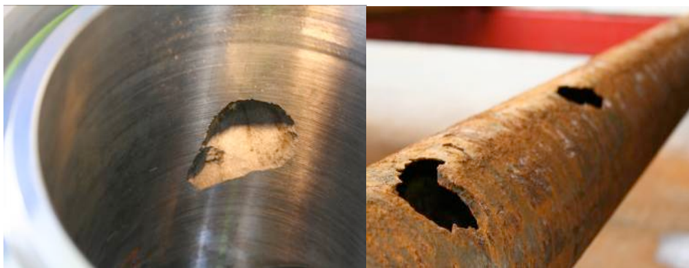
Figure 2. Illustrations of corrosion in of a well's tubing.
