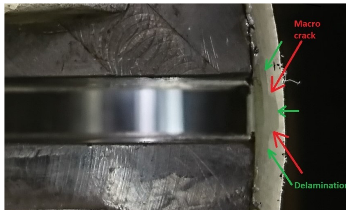
Figure 29. Macro cracks (red arrows) extending through the middle axial layer with delamination on either side of the middle axial layer (green arrows).
