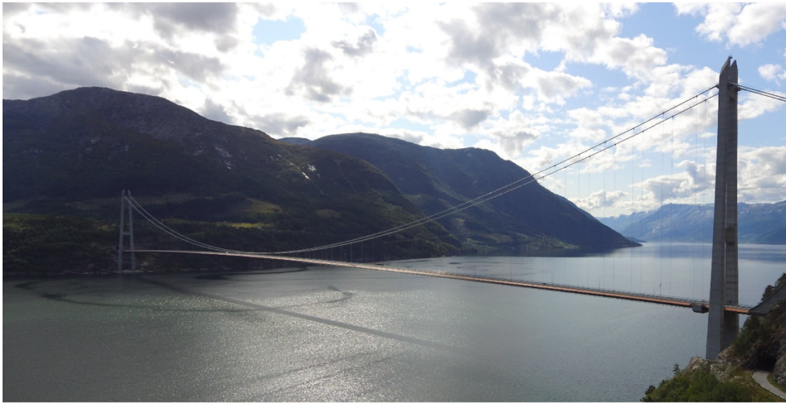
Fig. 2. The Hardanger Bridge seen from the northeast (picture by the authors).
