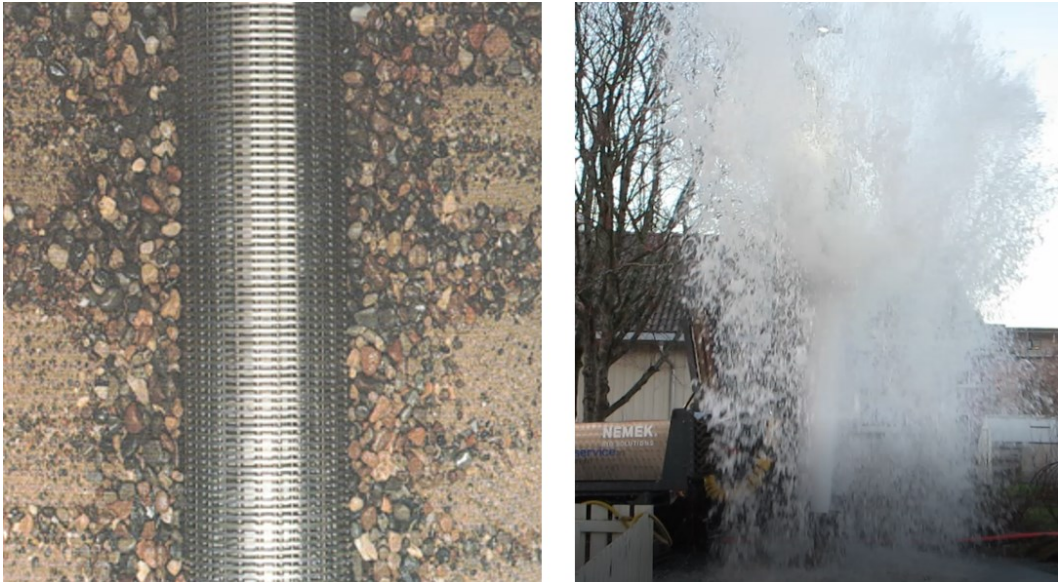
Figure 2: The left picture (from Driscoll) shows a con-slot well screen seen from the outside. A natural filter of coarser sand and gravel near the screen is made by washing (picture at the right) out the finer particles which can be seen further out in the formation. Washing of the well screen after installation can be seen of the picture to the right. Pulses of pumping air into the formation after the installation of the well screen, creates a “blow out” of water from the well. Many repetitions and sectionalized washing, ensures a well-functioning natural filter with high permeability around the well screen as seen in the picture to the left.
