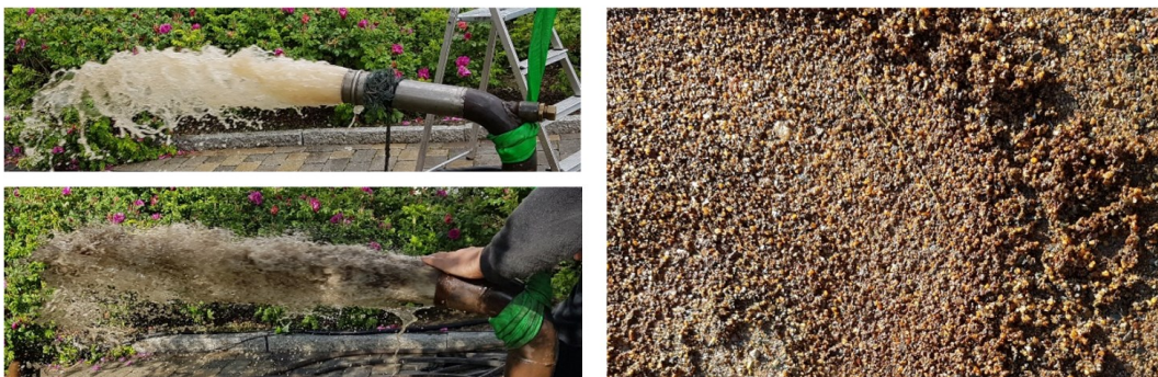
Figure 6: The pictures at the left shows the mammoth pumping in the upper and lower screen section, respectively. The upper picture is muddy water cleaning the aquifer formation outside the screen (inside the formation), while the lower picture shows very muddy water from removing the sediments in the lower part of the well. The picture to the right shows some of the removed material from the well. Note the reddish color.
