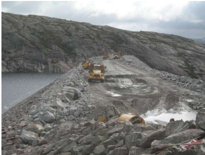
Figure 4. Dam crest during construction, Photo: Priska Hiller
