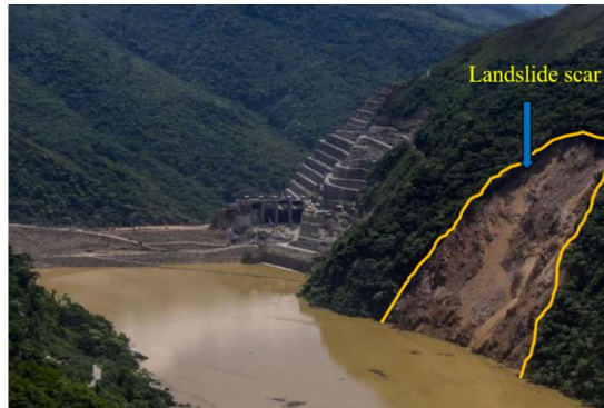
Figure 2: A large landslide scar at Hidroituango dam site, Colombia (Dave, 2018).
