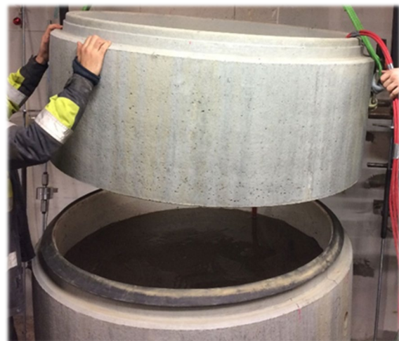
Figure 4.3. The chamber extension, note the rubber gasket on the rim of the chamber base.
