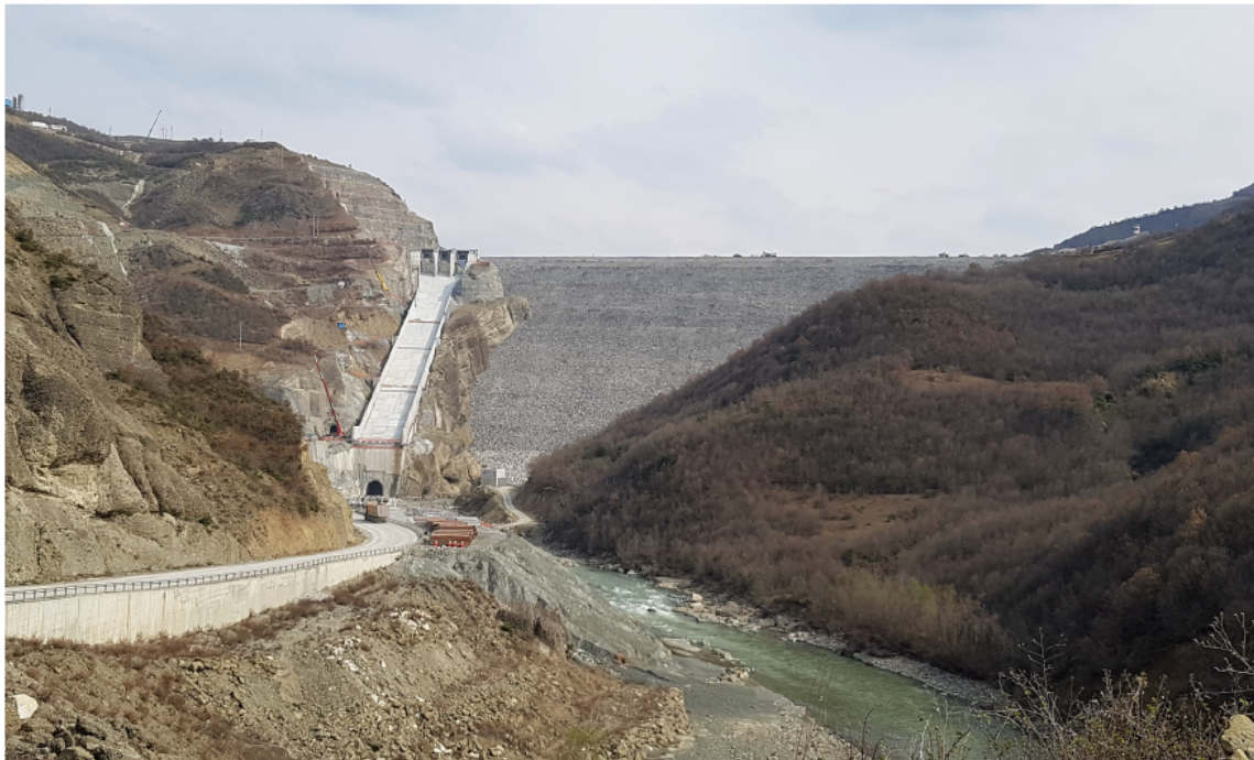
Figure 7.1: Moglice Hydropower Dam [Photo taken by Runa B. Frengen 27.03.2019 (Frenge, 2020)]
