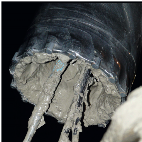
Figure 5.14: Drill casing after grouting in Dörverden.
