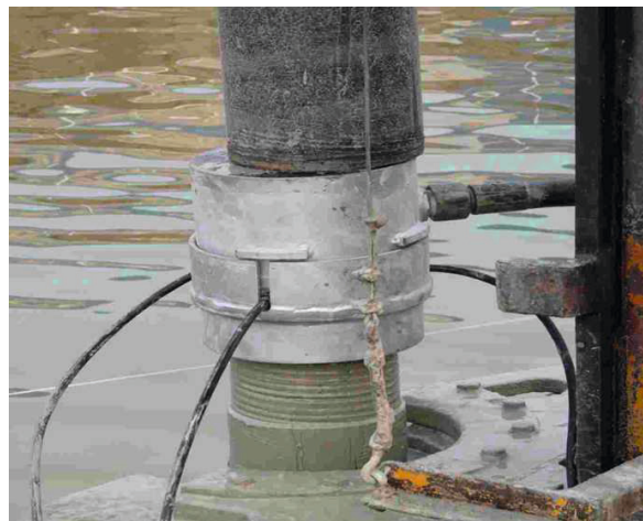
Figure 5.7: Modified grouting cap used to pump grout into the borehole in Dörverden.
