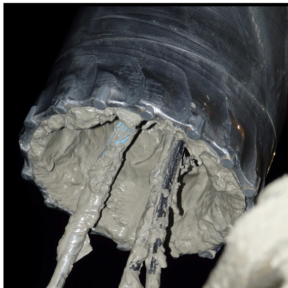
Figure 5.14: Drill casing after grouting in Dörverden.
