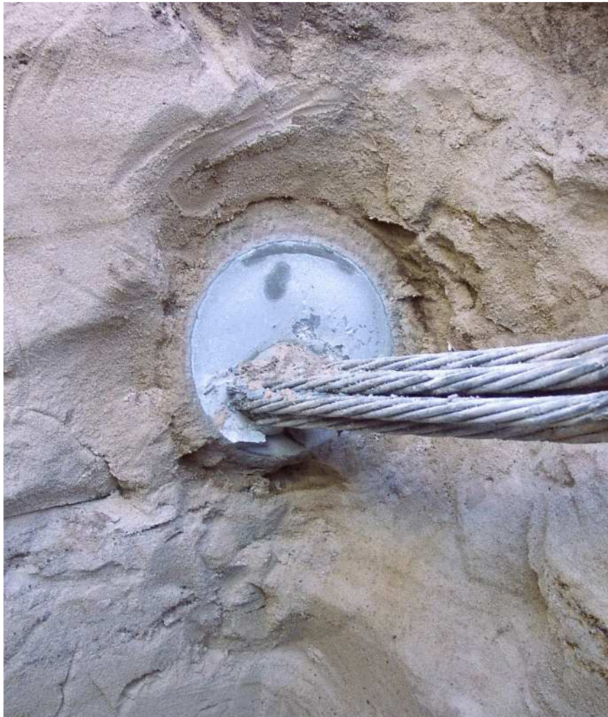
Figure 2.7: Exposed grout body in sand (by Brückner Grundbau GmbH).
