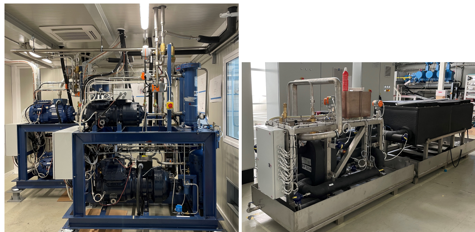
Figure 6. (left) Chiller room with two compressor slices and connections to gas coolers and common unit (right) Dummy load used to replicate operation of 2PACL system and heat load.
