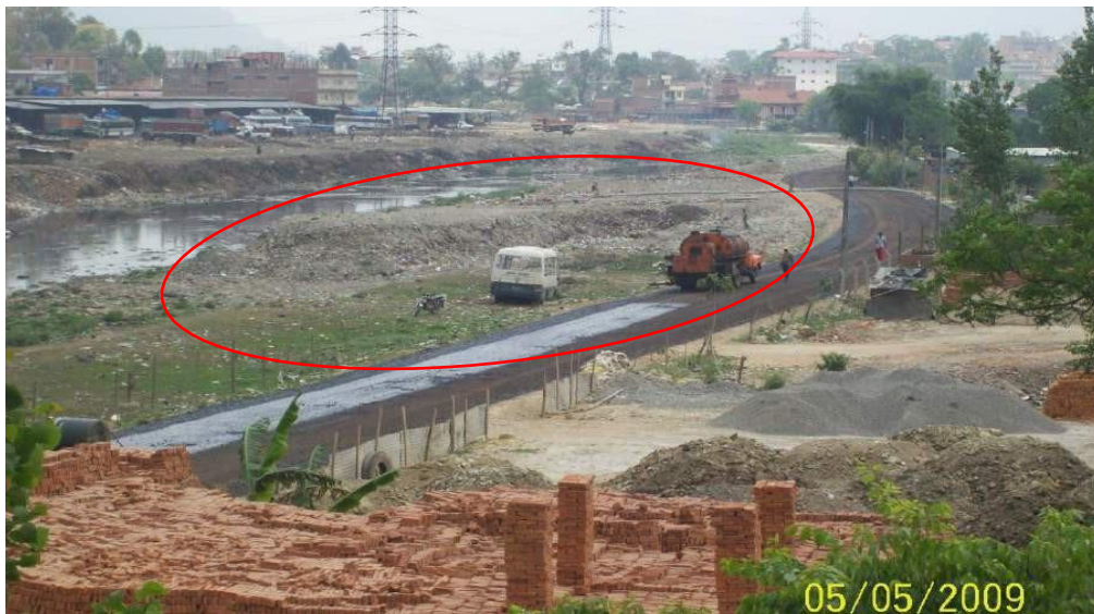
Figure 5-30 Garbage from encircled dumping ground being used for road layering (provided by Dr. Niva Baral)
