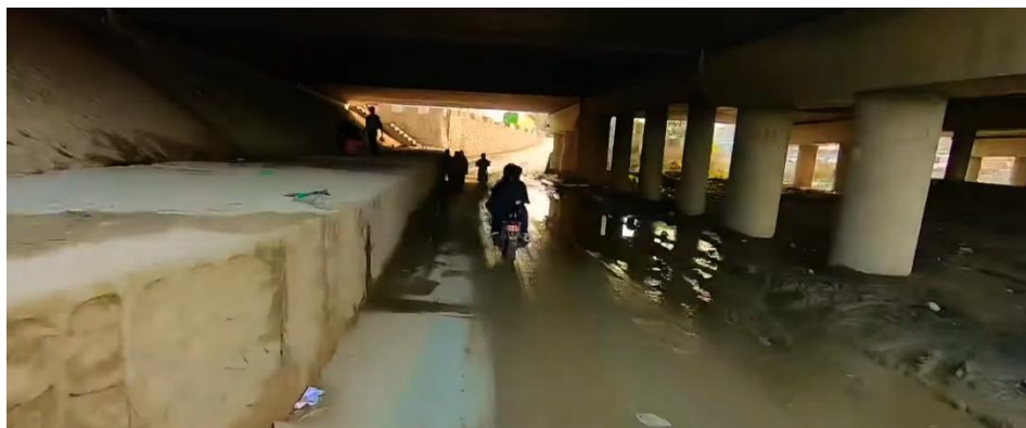
Figure 5-36 New road created underneath the Balkhu bridge (Ray4u, 2015)
