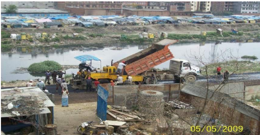
Figure 5-28 Road construction on Sanchal side in 2009 (provided by Dr. Niva Baral)
