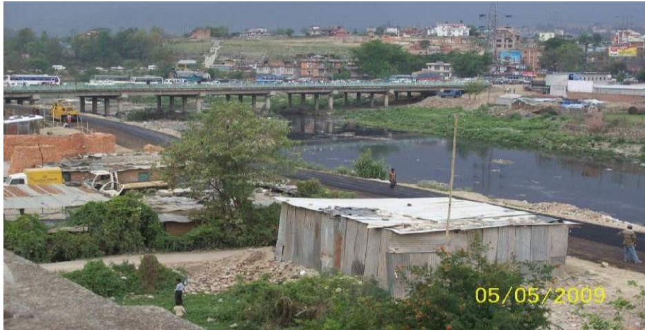
Figure 5-29 Road construction on Sanchal side in 2009 (provided by Dr. Niva Baral)
