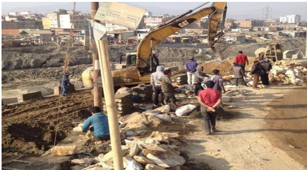
Figure 5-35 Ongoing path construction in 2015 (Dr. Niva Baral, 2015)
