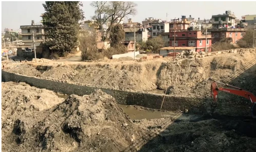
Figure 5-46 Stone retaining wall construction in case study area in 2019 (Ray4u, 2019)
