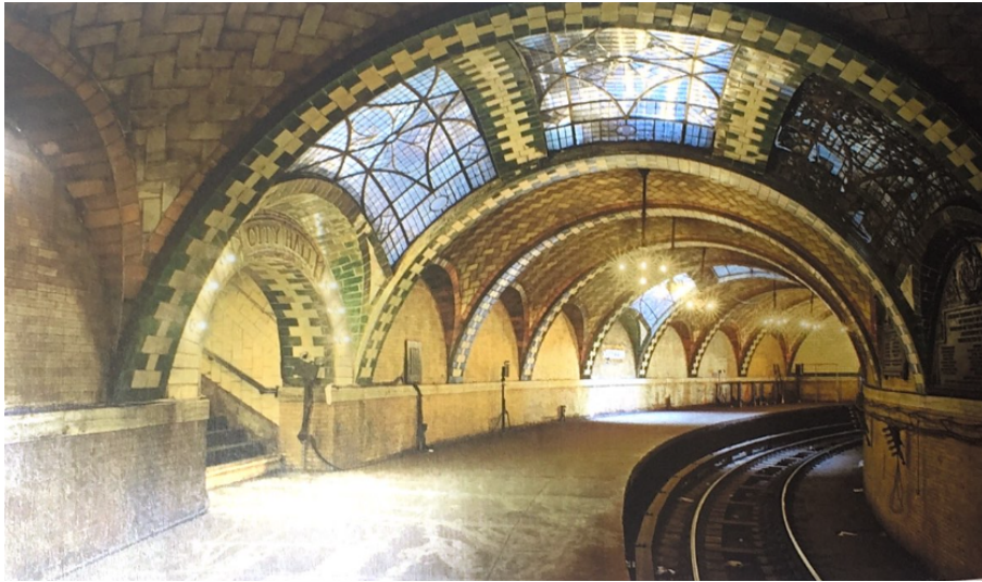
Figure 10: City Hall Subway Station, tile vaulting
