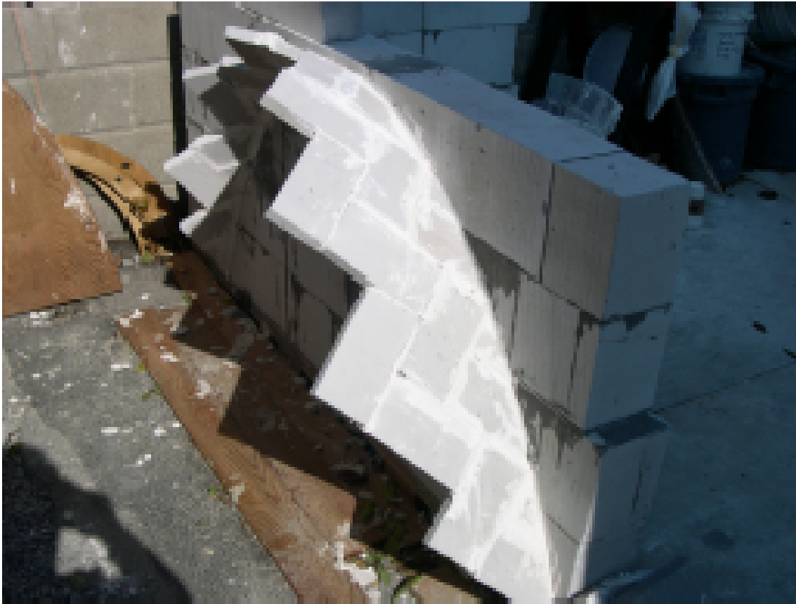
Figure 43: Cantilevered barrel vault
