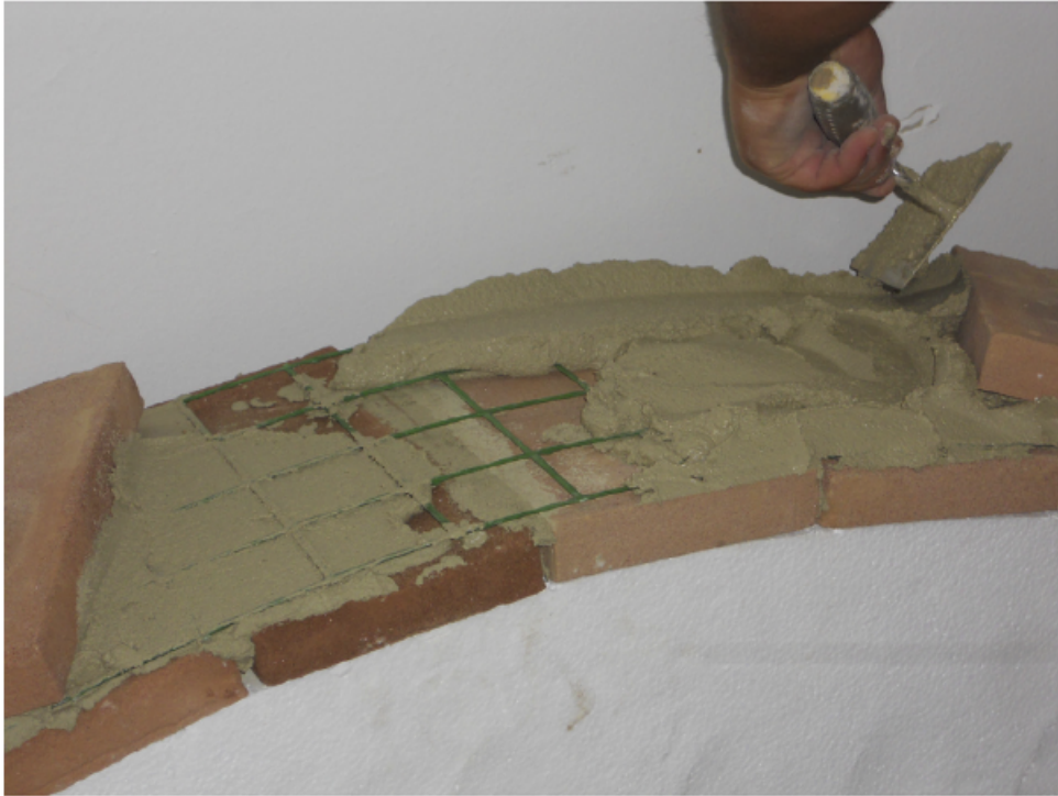
Figure 63: Application of GFRP grid
