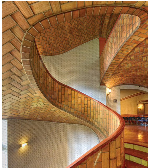
Figure 14: Tile vaulted staircase of Baker Hall, Carnegie Mellon University, Pittsburg, 1914
