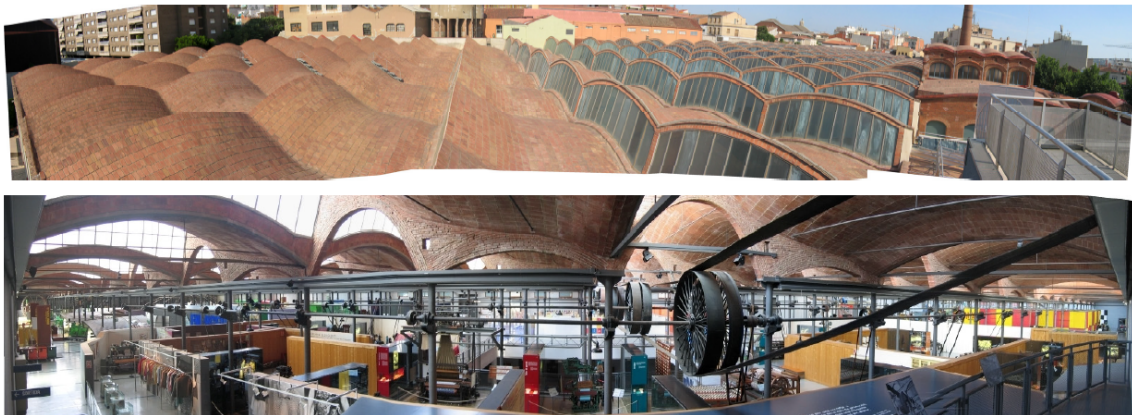
Figure 5: Roof and interior of Aymerich, Amat i Jover textile factory
