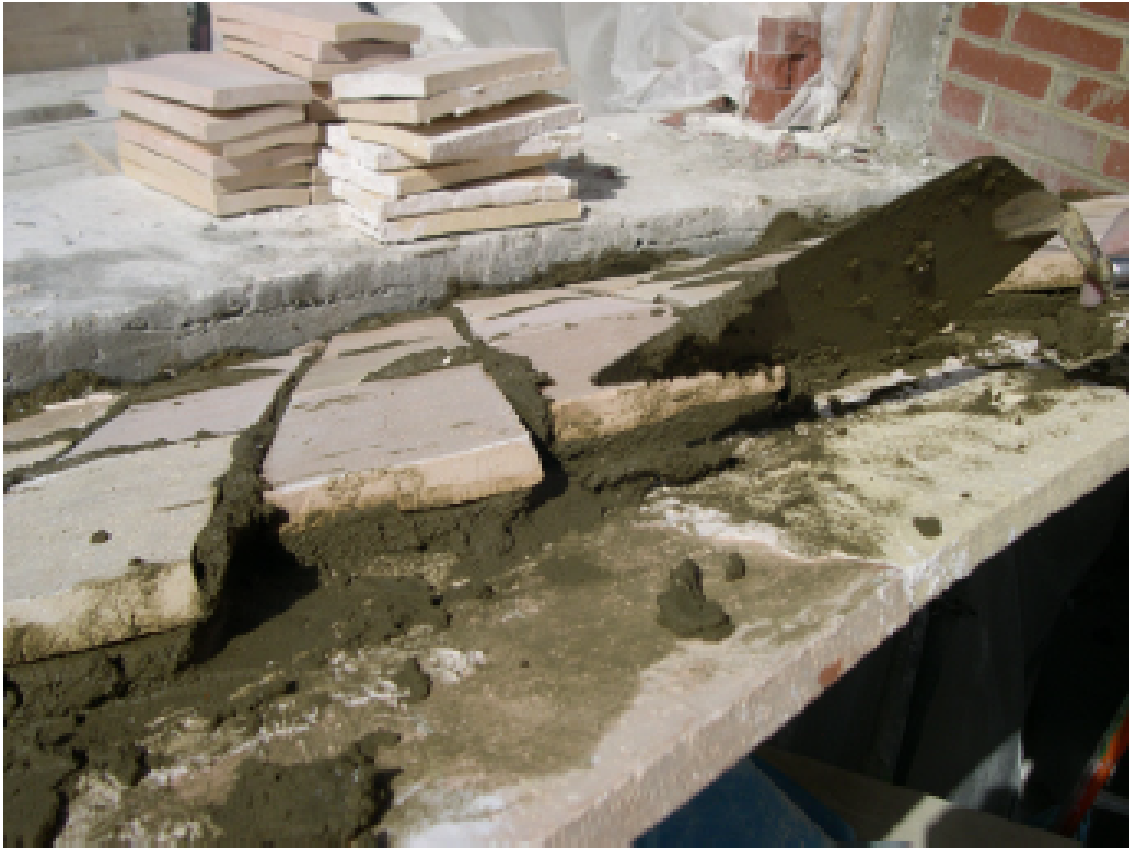
Figure 57: The second layer mortar bed
