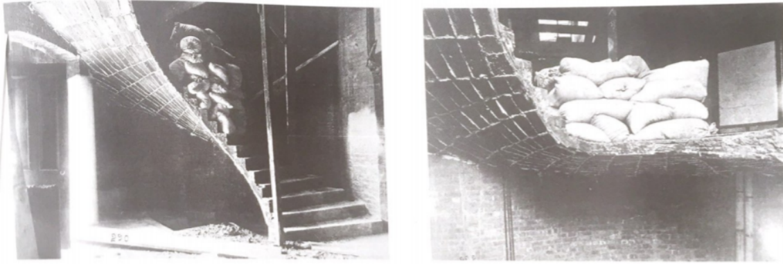
Figure 9: Load test on a Gustavino helicoidal tile stair, first Church of Christ Scientist New York City, ca 1900
