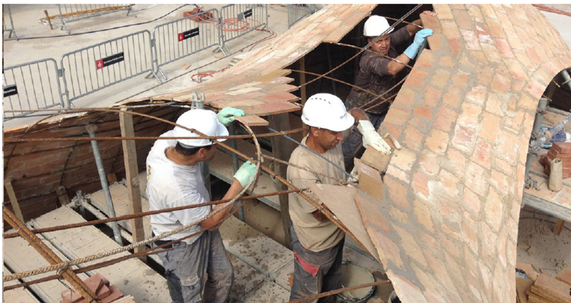
Figure 51: Another system for falsework
