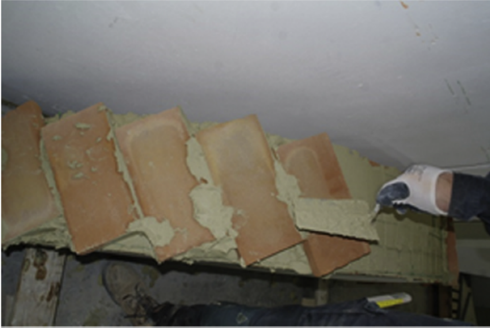
Figure 64: Application of the second layer of flat tiles
