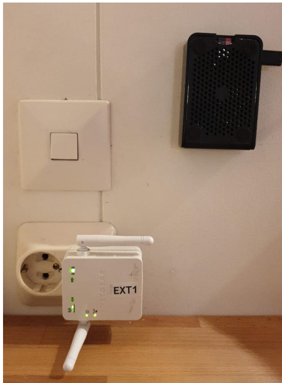
Figure 6.3: Photo of the Raspberry Pi, which is the black device hanging on the wall, and the Wi-Fi router, which is the white device.
