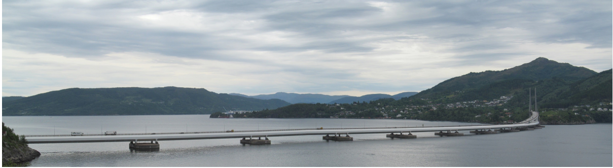
(a) The Nordhordland Bridge (European Roads, 2014).
