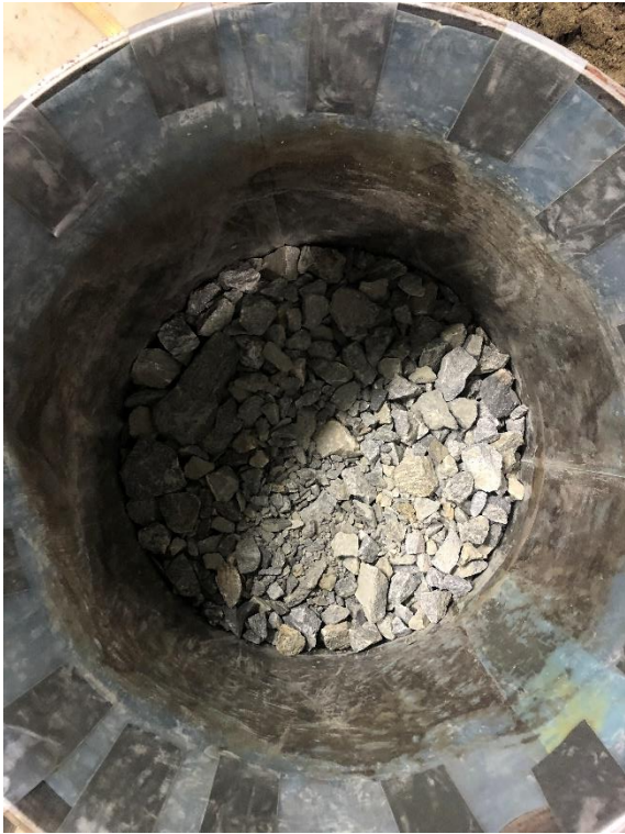
Figure 0.49 CR 1, first layer, compacted
