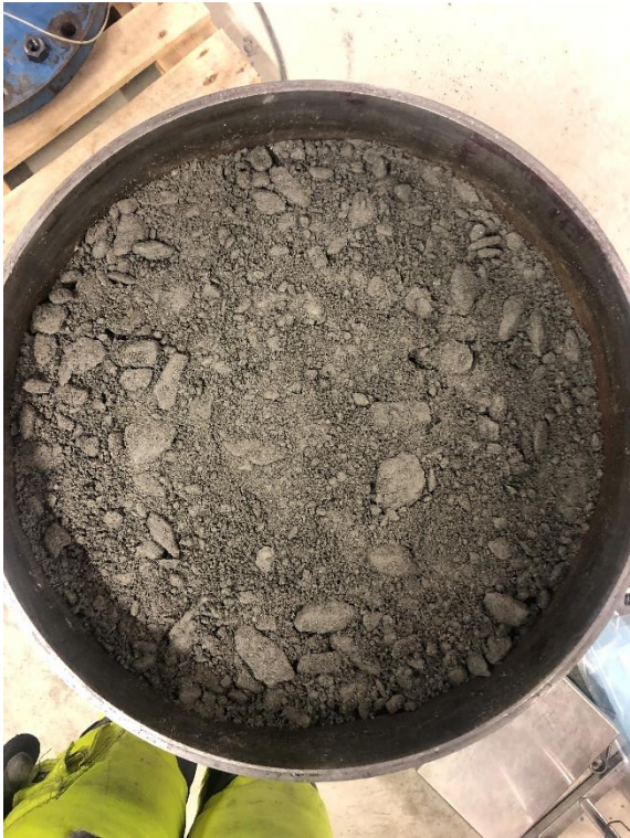
Figure 0.45 TBM 4, fifth layer, compacted
