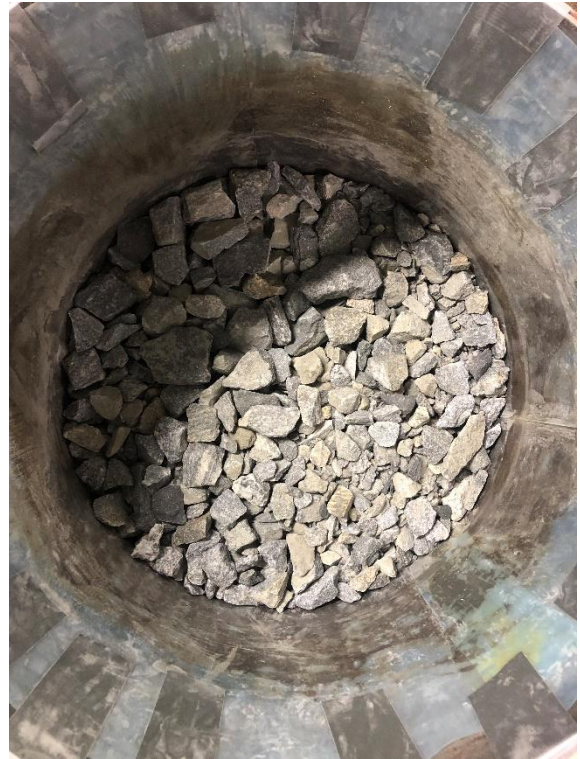
Figure 0.46 CR 1, second layer, compacted
