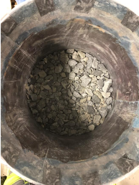
Figure 0.62 CR 3, first layer, compacted
