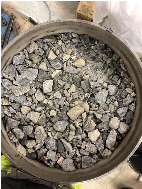
Figure 0.58 CR 2, fifth layer, compacted
