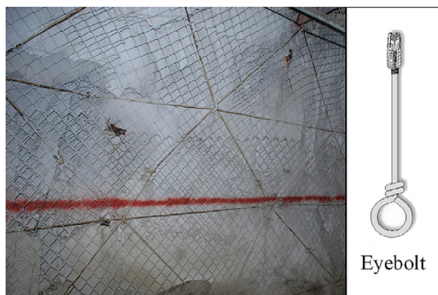
Fig. 25. Lacing on the wall of a deep mine drift in South Africa.
