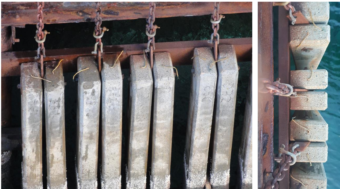
Figure 4: Concrete beams (concrete P, E, B and D from left to right) mounted from the ferry quay at the Field Station Sandnessjøen (14 th March.2018 – Photo: Tobias Danner)
