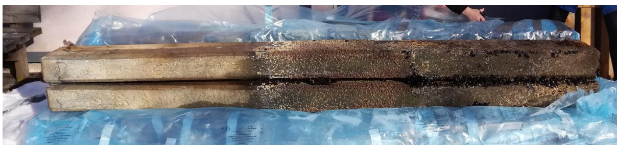
Figure 10: Pair of loaded concrete beams as received at NTNU before cleaning the surface, submerged part of the beam to the right (15 th March 2018 – Photo: Ragnhild Moastuen)
