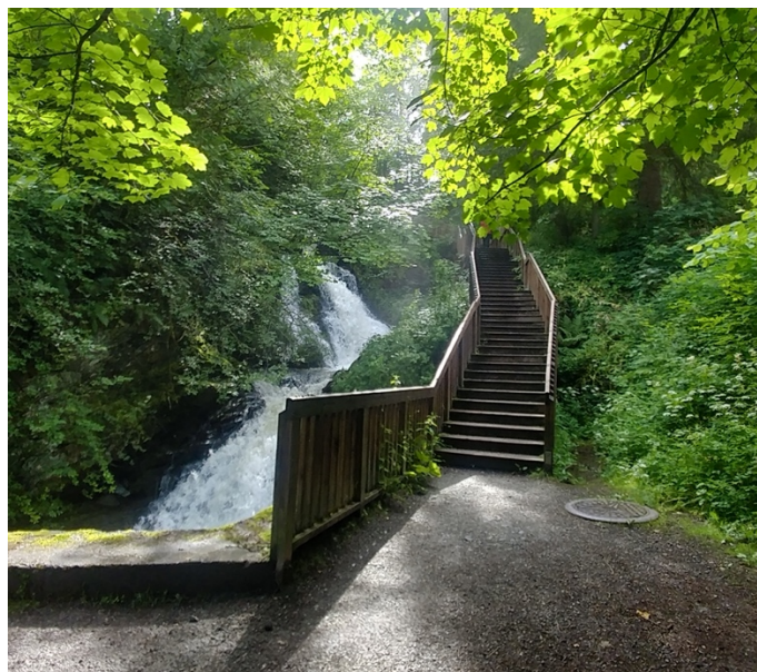
Figure 5.17 Wooden stairs with temporary structure to not intervene with the geographically valuable rocks (Source: Author)
