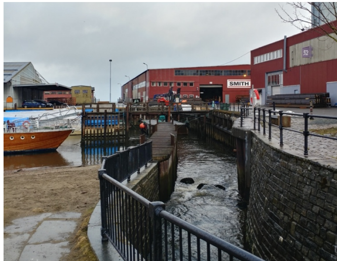
Figure 5.18 A mixing system in the water to not let the fresh water from the stream to be released to the fjord, causing icy surface in the winter time (Source: Author)
