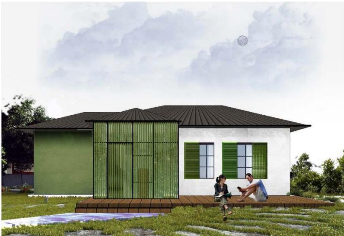
Figure 5-6. Facade view of the housing typology. (Construction company, Commonsense Architecture Studio, 2020)
