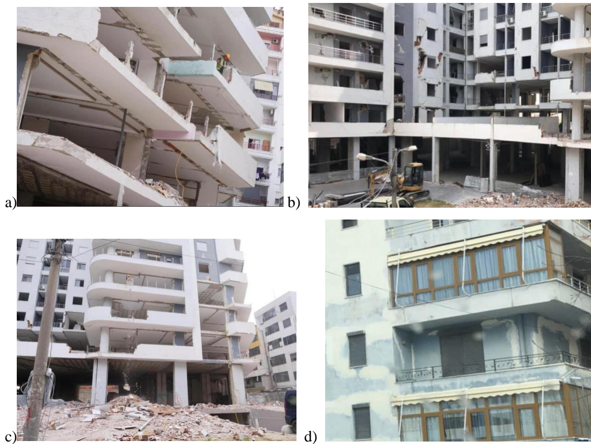
Figure 5-7. Process of building retrofitting in Durres city. (By the author)
