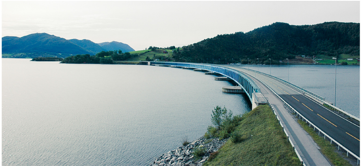
(b) The Bergsøysund Bridge (Kvåle, 2017).
