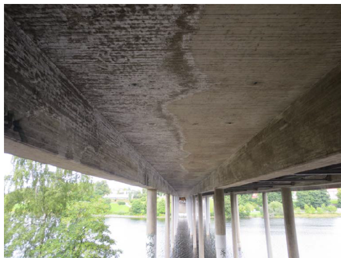
Figure 3.5: Moist concrete in plate between inner and outer beams [16]
