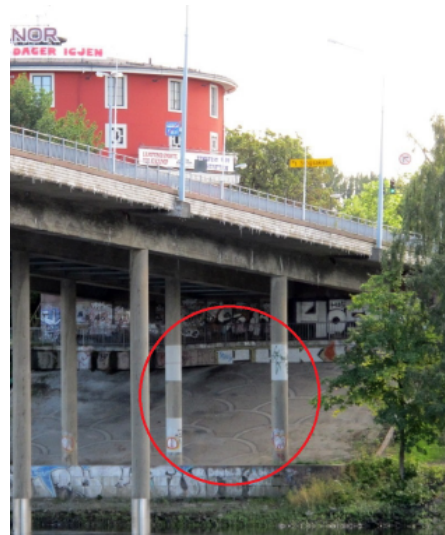
Figure 3.9: CFRP on columns A and B in axis 2 [18]
