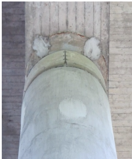
Figure 3.8: Column top in axis 9 after correction [18]
