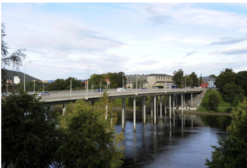
Figure 3.1: Elgeseter Bridge seen from the east [12]
