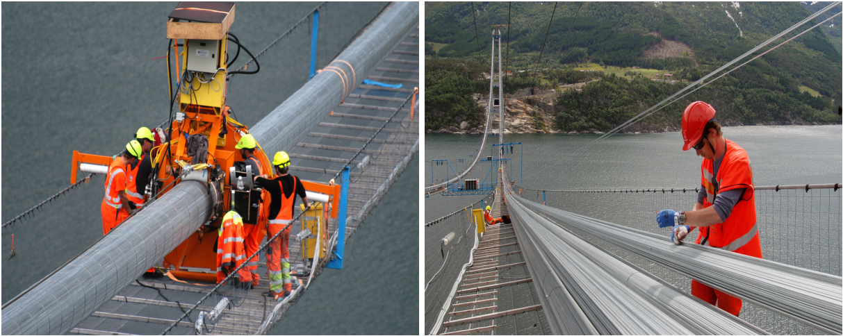
Figure 3.4: Assembly of the main cable. Photo: Statens Vegvesen [12]
