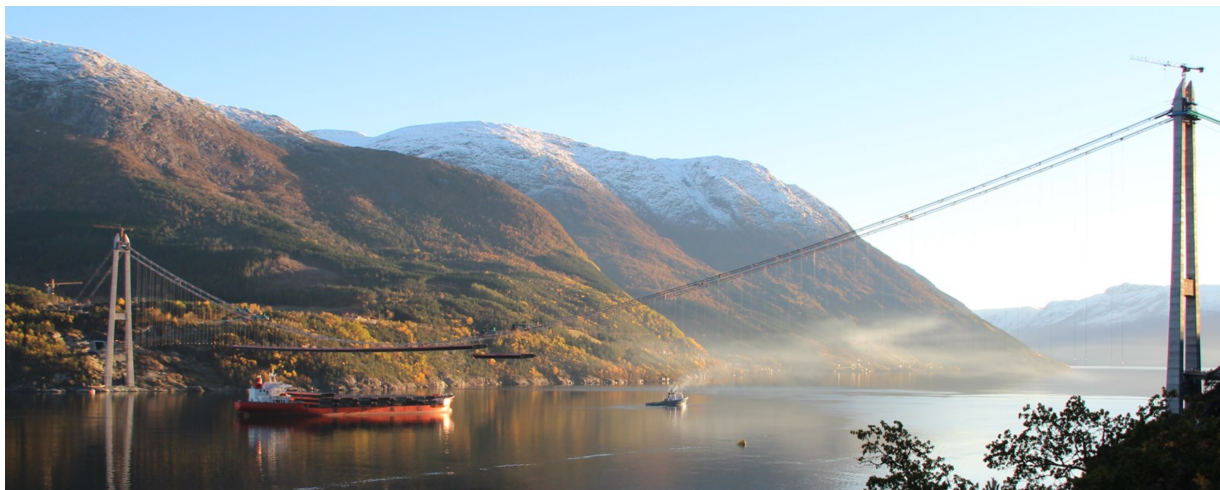
Figure 6.1: Assembly of the stiffening girder. Photo: Norconsult [35]
