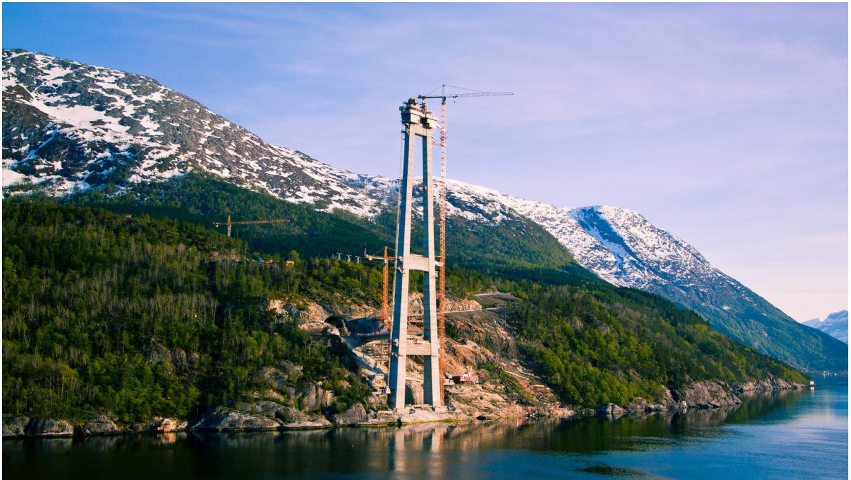
Figure 5.1: Southern bridge tower of Hardangerbrua. Photo: Roth T. [32]
