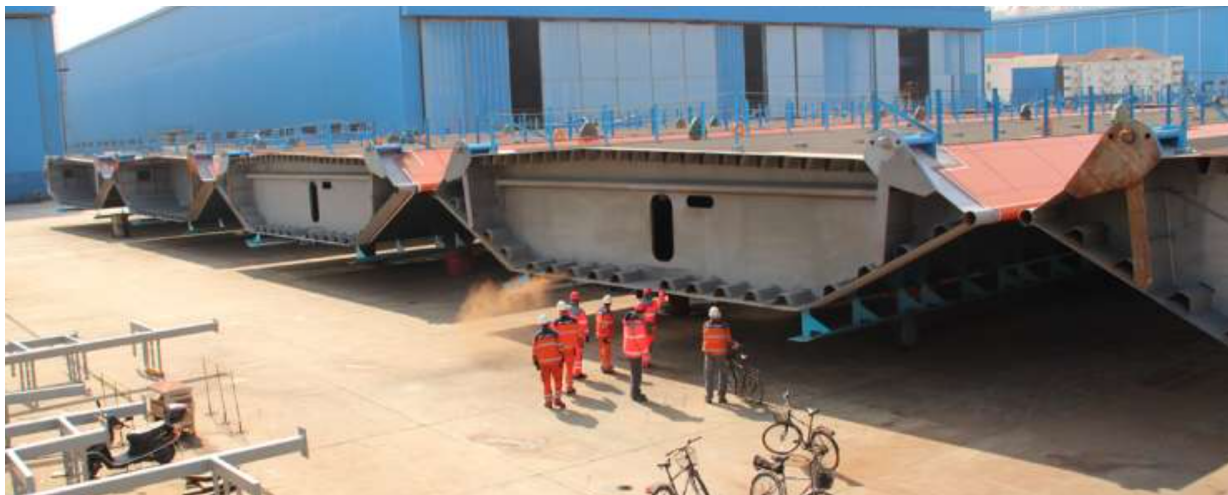
Figure 2.5: The stiffening girder of Hardangerbrua. Photo: Statens Vegvesen [3]
