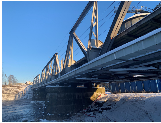
Figure 4.3: Picture of Sokna Bridge.
