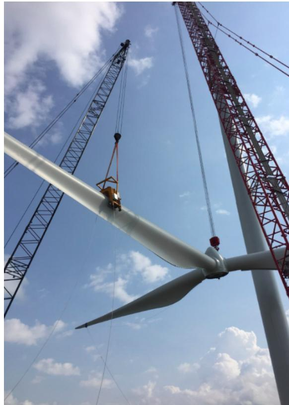
The mounting of hub and blades will be the most complex and time demanding operation in the whole process. The sweeping area of blades will be significant large, and therefore requires calm weather.
