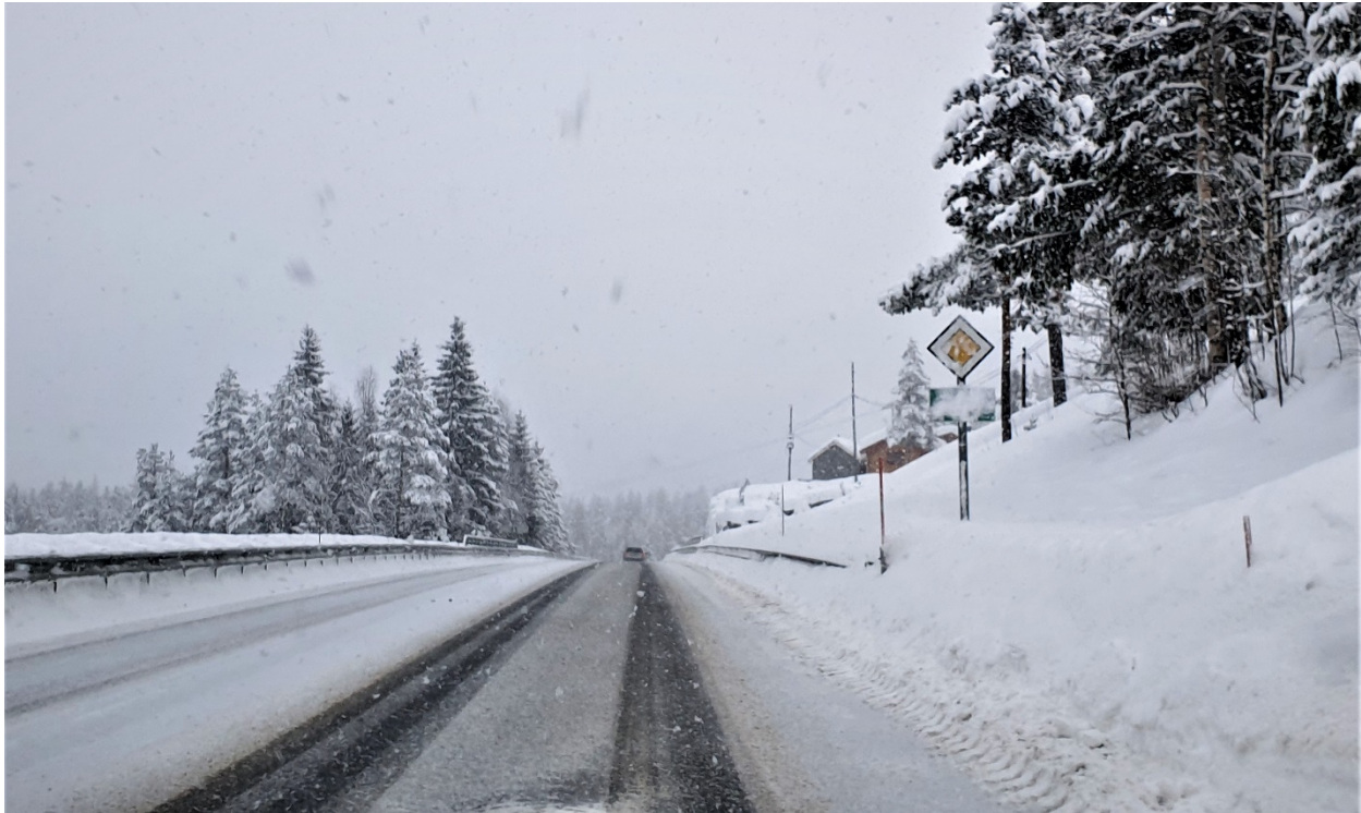
2 FIGURE 2: Road conditions that are probably unsuitable for automated vehicles, where road signs and 3 lane markings are covered with snow. E16 in Valdres, Norway. Photo: Ingvild Ødegård 4 5
