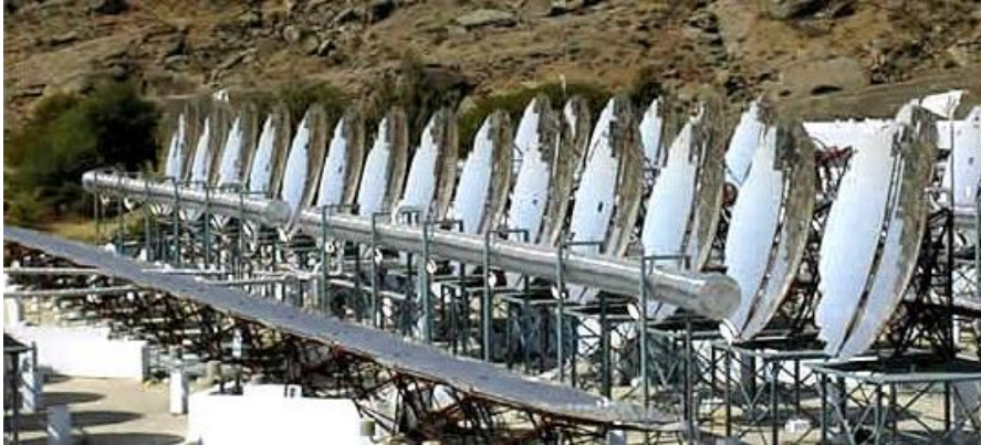
Figure 1.9: World's largest steam based indirect solar cooker [22]
