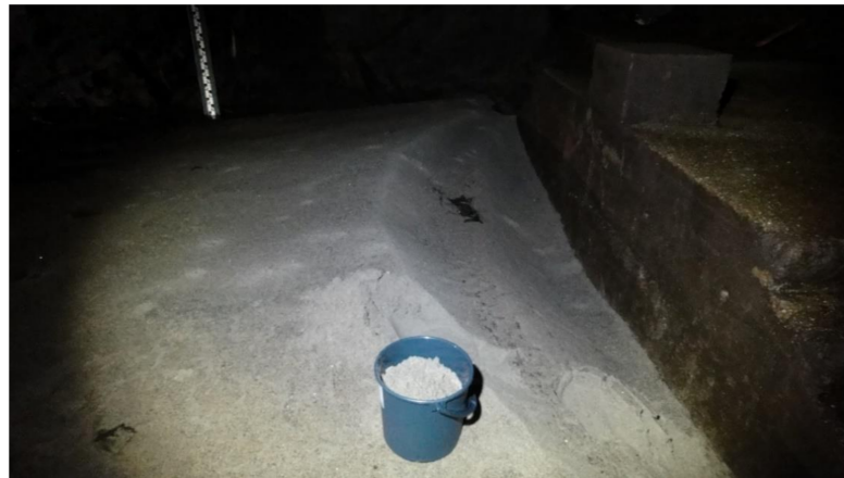
Figure 5. Picture of sediment deposited before the weir in the downstream end of a pressurized rock trap at the 960 MW Tonstad hydropower plant, Norway. Flow direction from left to right.
