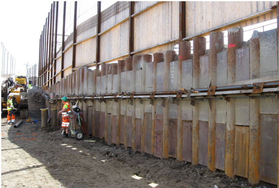
Figure 4.2.2: Pile wall for construction of Nordenga bridge, from Geovita AS.
