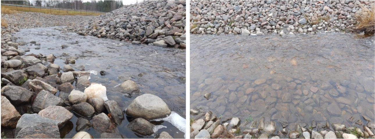
Figure 5.12 Pictures of the rearranged part of Stabekken. The stones in the side slopes (left pictures) and on the bottom (right pictures) of the stream can be seen in the pictures (Photos by: Kristine Bergseng).
