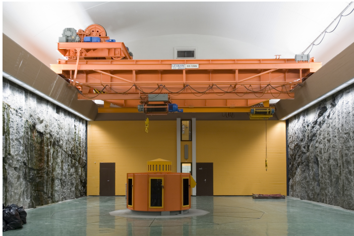
Figure 1.2: The Roskrepp power plant [2]
