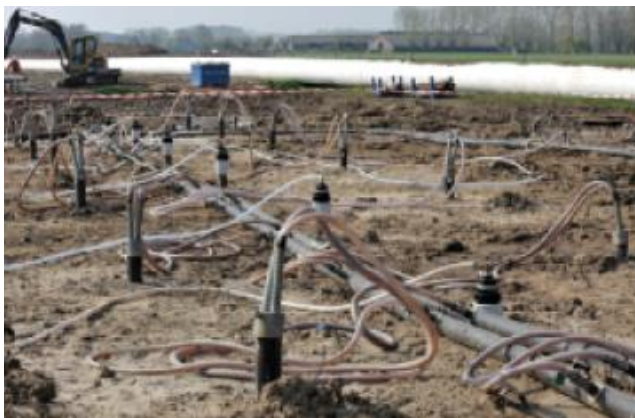
Figur 101. Show grid of injection wells on top of projected pathway for pipeline (left) and stabilized gravel (right). Images from (Van der Star et al., 2011) (left) and (DeJong et al., 2014) (right)..
