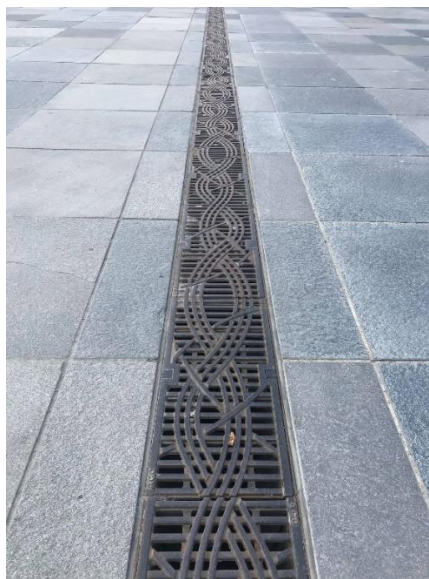
Figure 7: Photo of a part of a long gutter stretching across the square.
