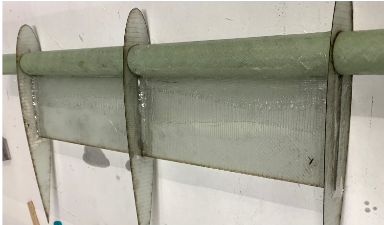
Figure 5.14: The rudder stock and spokes during adhesive bonding.
