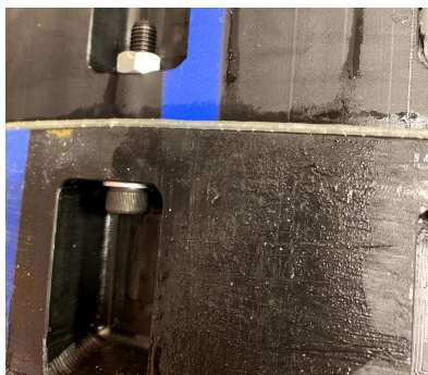
Figure 6.2: Joint 3 under waterproof test.
