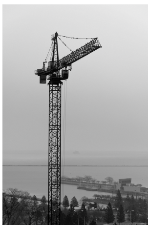
(a) Tower Crane.
