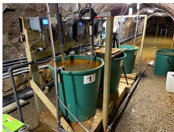
Figure 2.2 The tunnel with Trondheim municipality's system in January 2019. The system changed over time. For more information about the changes made in Trondheim municipality's system, see appendix A.
