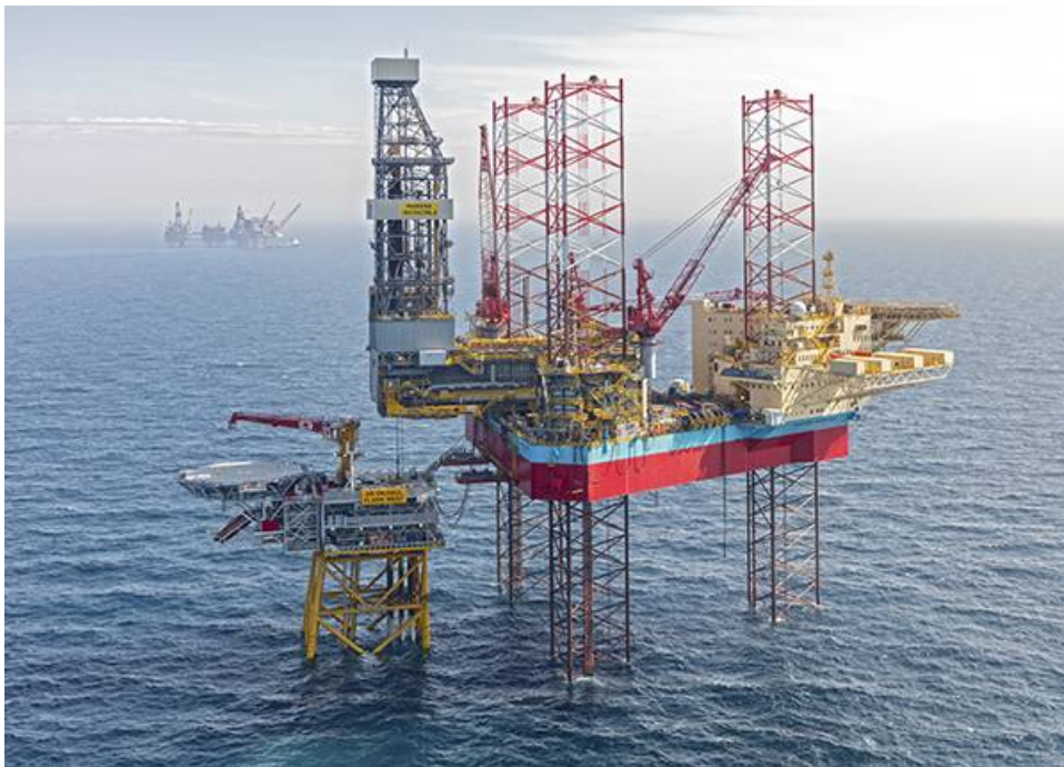
Figure 5: Typical jack-up rig design (Offshore 2020)
