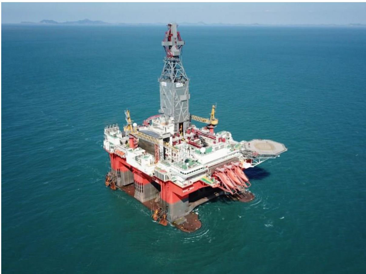
Figur 1. West Mira rig (Offshore Energy, 2018)
