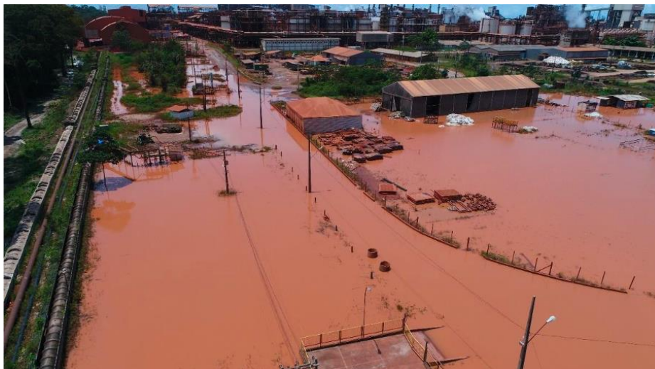
Figure 7 Area 45 at Alunorte flooded after the heavy rainfall in February 2018 13 .
