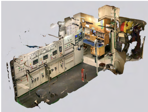
(e) LiDAR scan of the model explored in the Outside Engine Room, i.e. control room scene.
