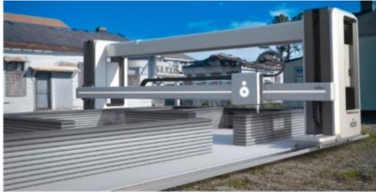
Figur 22: ICON's printer i drift i Austin Texas (Souza et al., 2020)
