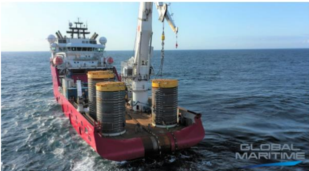
Figure 37 – Suction anchor installation (Global Maritime, 2019).
